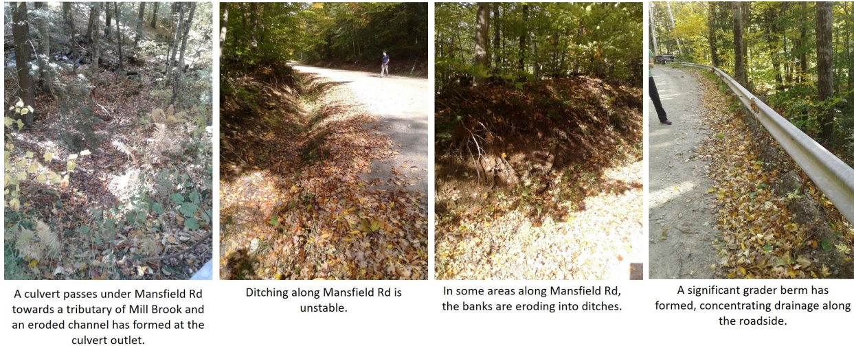
Figure B21. The proposed retrofits are described in the above photos.
