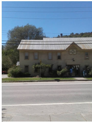
Figure C13. Proposed subsurface sand filter is located under the Post Office parking lot.
