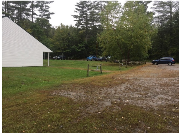
Figure B13. Drainage from the Town Office parking lot is currently unmanaged.
