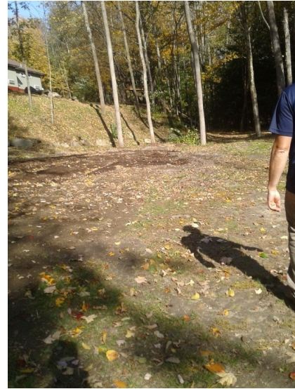
Figure E12. A bioretention practice is proposed in the low spot pictured in the middle left side of photo.
