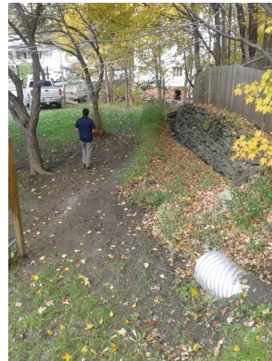
Figure E11. Step pools are proposed between the culvert outlet pictured above and river.
