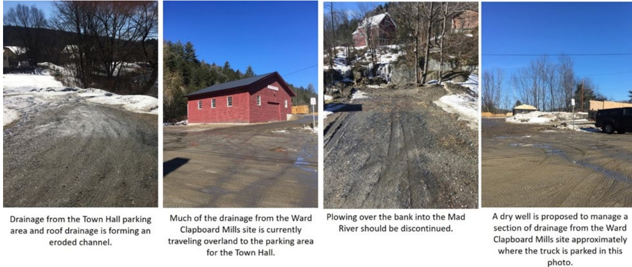
Figure C23. The proposed retrofits are described in the above photos.
