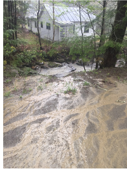
Figure B10. Stormwater is running over road directly to stream and transporting sediment.
