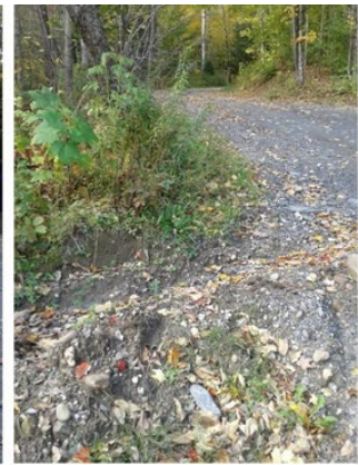
Areas where runoff is eroding areas along the access road. The area (pictured left) is the proposed location of a new culvert and level spreader.
