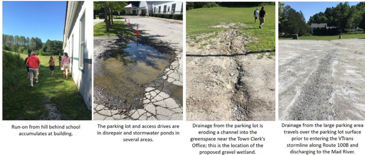
Figure C19. The proposed retrofits are described in the above photos.
