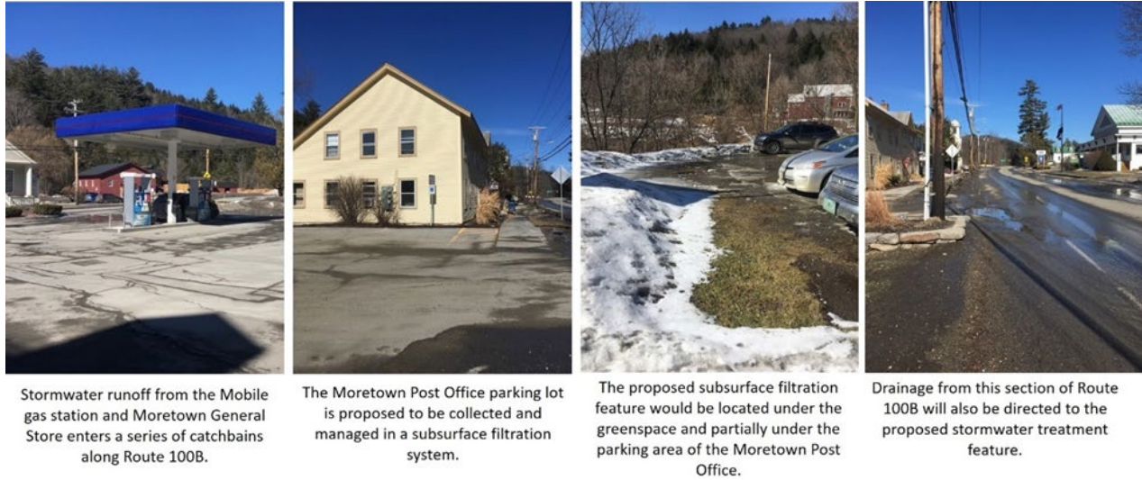
Figure C25. The proposed retrofits are described in the above photos.
