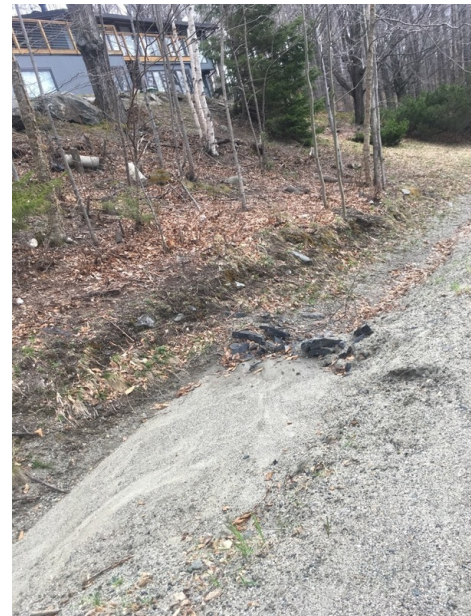
Figure E9. There are issues with sediment transport along Slopeside Development’s private roads.
