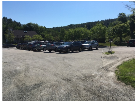
Figure C10. It is proposed that the drainage from the Moretown Elementary parking lot be managed in a gravel wetland.
