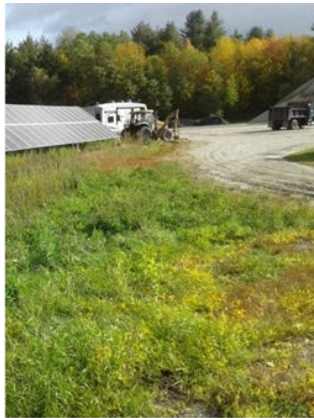
Most of the site drains to this swale by the solar panels.
