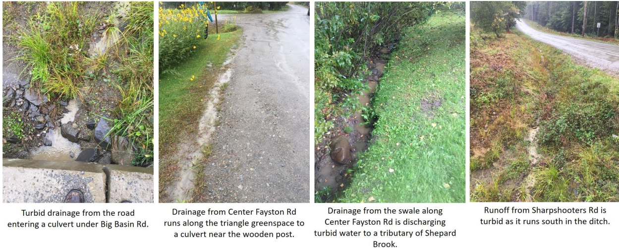
Figure B23. The proposed retrofits are described in the above photos.
