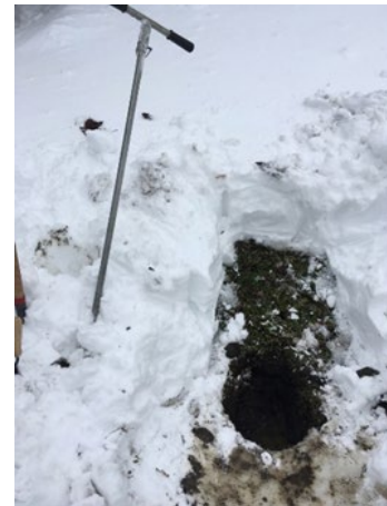
Figure E16. Soils were assessed in the roadside ditch area.
