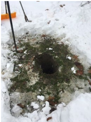
Figure D30. A hand auger and shovel were used to assess soil conditions and infiltration potential.
