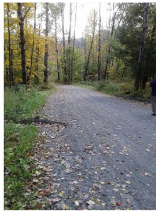
Areas where runoff is eroding areas along the access road. The area (pictured left) is the proposed location of a new culvert and level spreader.
