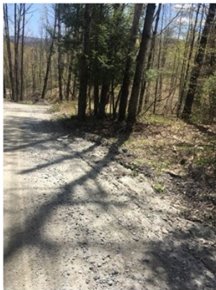
Water currently runs down the Town gravel pit’s access drive towards Vaughn Brown Rd and VT-100. An infiltration basin is proposed just northwest of the intersection of the access road and Vaughn Brown Rd to collect and infiltrate runoff from the road.
